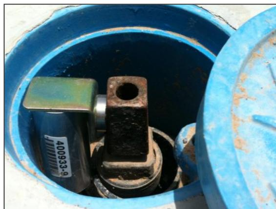
Figure 1.4 Acoustic logger deployed on a valve spindle with a bracket
