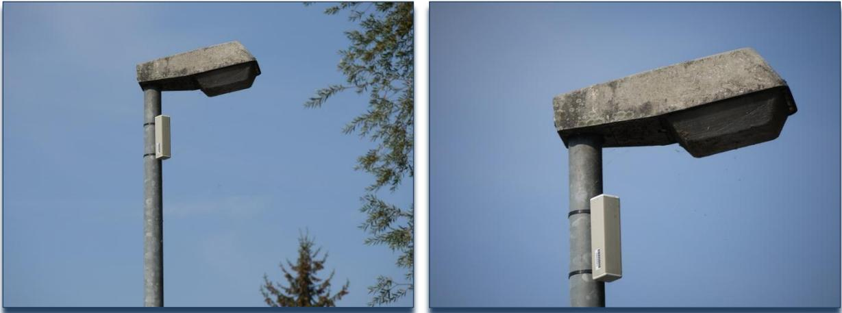
*Figure 2 shows REPEATER set on a lamp post*
